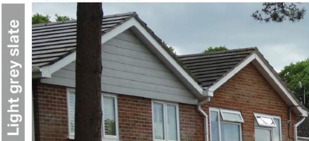
Double gable roof sharing the same roof materials and colours.
