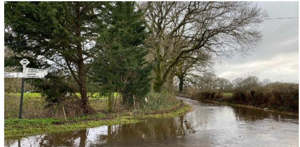
Figure 2. Local flooding (Harbridge Drove / Ringwood Road)
