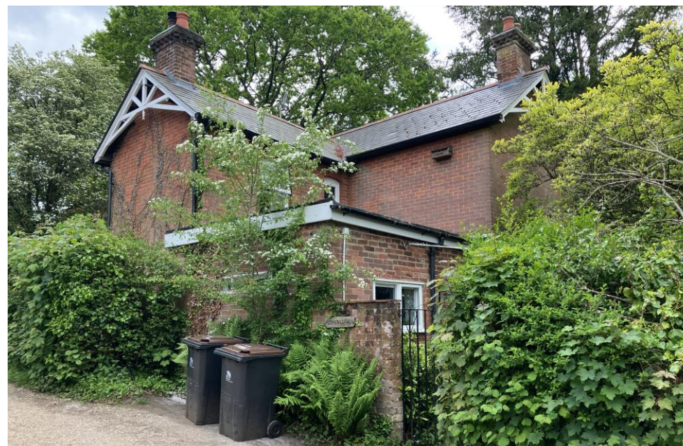
Figure 13. Decorative gable end, ridge tiles and chimneys
