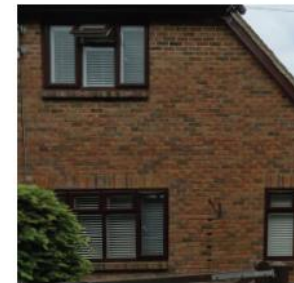
Dark wood frame casement windows.
