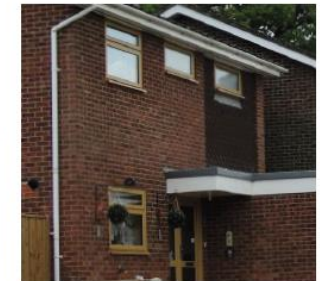
Timber framed windows and doorway.
