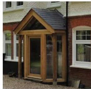
Gable portico with timber frame and glazing.
