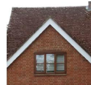
Timber casement window with arched brick lintel aligned under gable.
