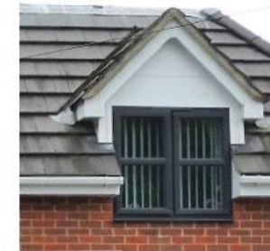
Gable dormer with painted timber casement window.
