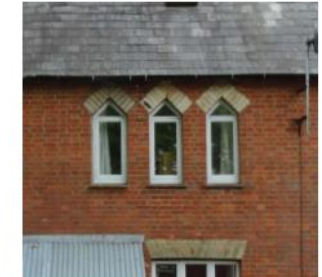
Brick lintel detailing above fenestration.
