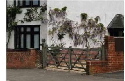
Low brick wall with timber entrance gate.
