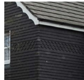
Continuous pattern in weatherboards and decorative fascias.
